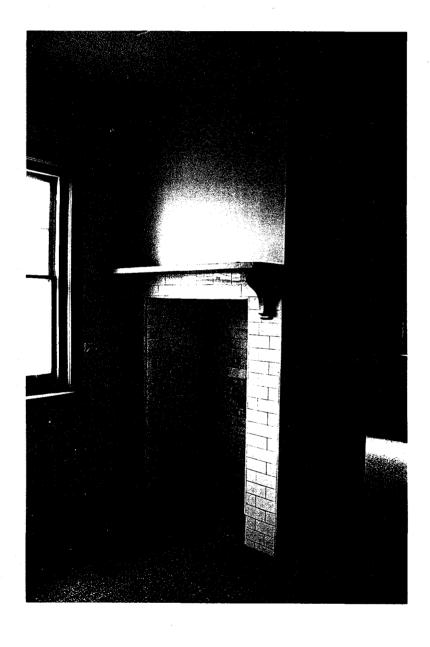
Figure 41 Building 9. First floor flat, showing tiled stove recess in kitchen.
