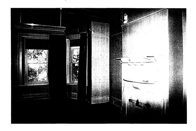
Figure 49 Building 10. East wing, Ground floor room 327, showing nineteenth century pressed metal ceiling and c. 1920 mantel.
