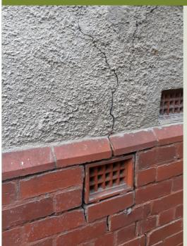
Cracks in one of the older-style buildings: evidence of underlying structural damage that requires priority attention.
