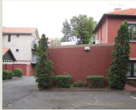
Maintenance building (north wall) now
